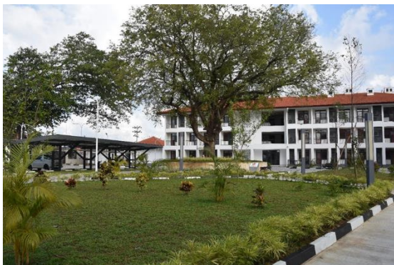
Figure 03: Accommodations area - National Nephrology Specialized Hospital Polonnaruwa - 2022
